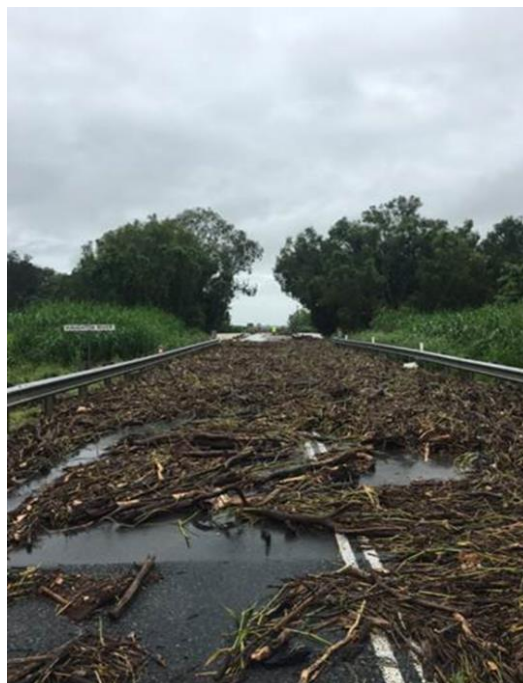
Figure 2. Flood debris across the Bruce Highway at the approach to the Haughton River bridge (credit: Queensland Department of Transport and Main Roads).
