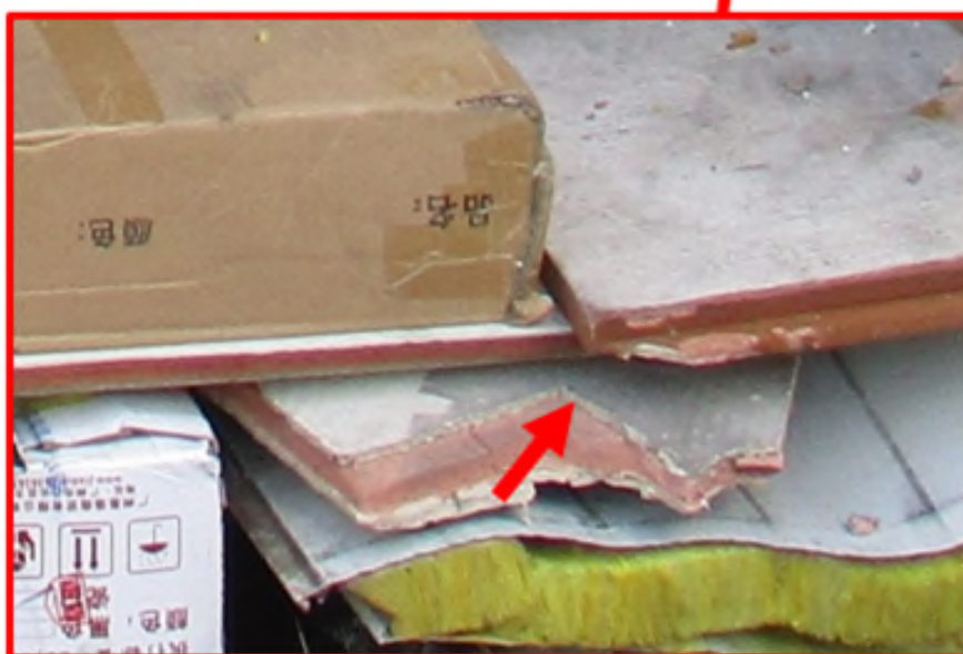
Arrow indicates outer section of cement fibre board containing asbestos.
