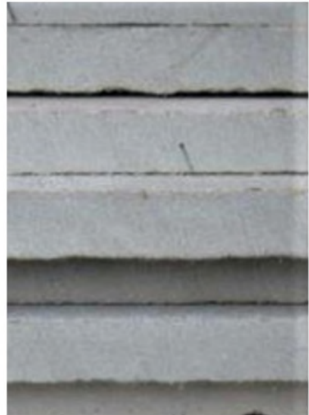
Boards visibly contain fibre material
